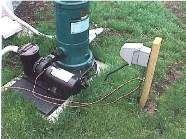
The bond wire shall be a solid #8 copper wire coming from the pump motor to the rigid metal conduit picking up pool heater if applicable. The pool must also be picked up by the bond wire. Check upper and lower rings- if they are metal, they must be picked up by the solid #8 wire. This can be achieved by inserting solder-less lugs where screws hold uprights and rings into place.
