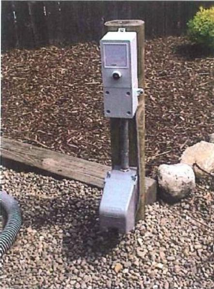
Pool light must be hardwired. Check your pool light box for splice box and manufacturer's installation instructions. Note: You must obtain a 6-8" rigid electrical pipe nipple to go between the outlet box and splice box of the pool light.
